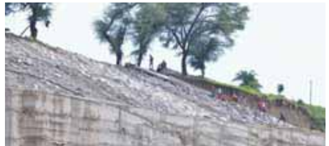
Construction of retaining wall at Baneshwar anicut to protect villages from diversified flow of water
